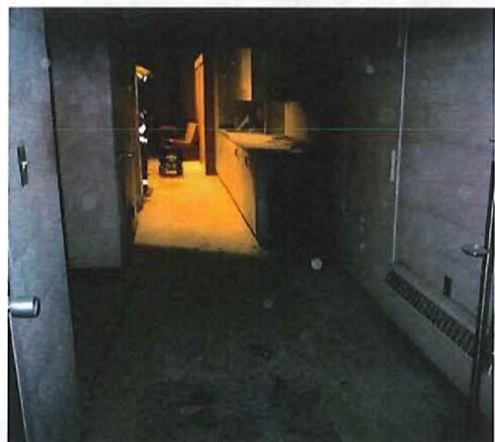
Fire at Our Lady of Sorrows Church
