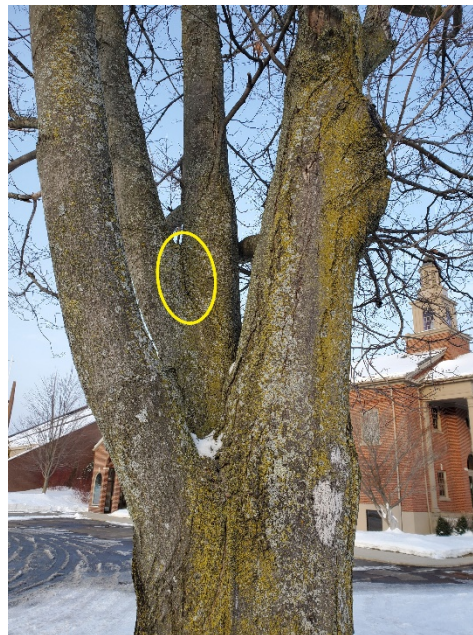
Poor branch attachment that would have been easier to correct when the tree was smaller.
