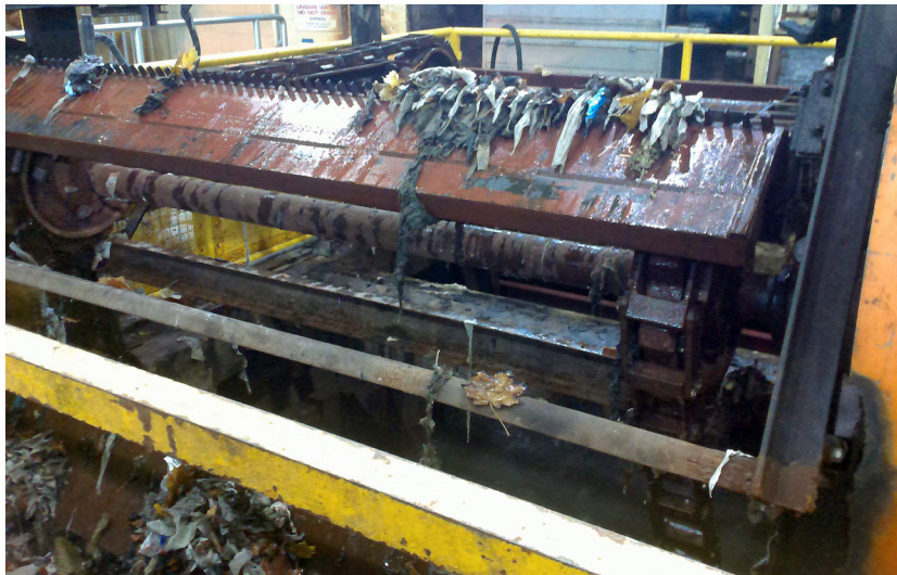
Nonwoven wipes clog sewers and equipment in pump stations and wastewater treatment plants because they don't break apart in water. The extra maintenance required to remove them comes at a cost to all sewer system users.
