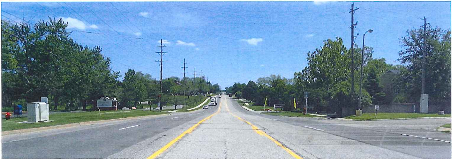
CS 63821/63022, JN125583 Grand River Avenue (Old I-96) from 8 Mile Road to 10 Mile Road Metro Region Roadway Scoping
