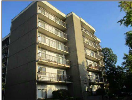
20. Side building elevation (east) facing northwest.
