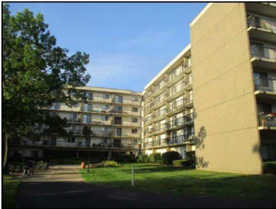
19. Back building elevation (east and north) facing south.
