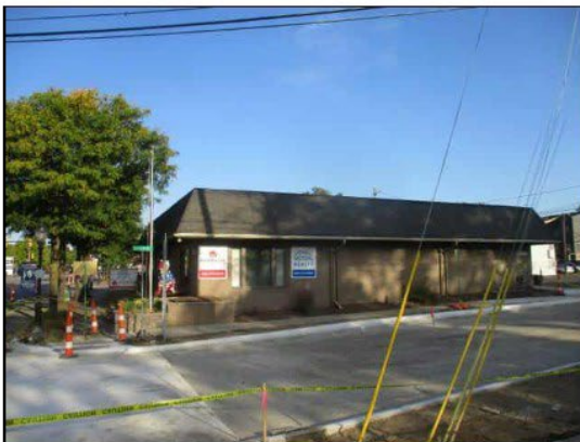
65. West adjoining office building (33004 Grand River Avenue)
