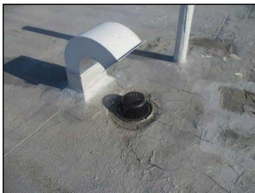
49. Typical roof drain
