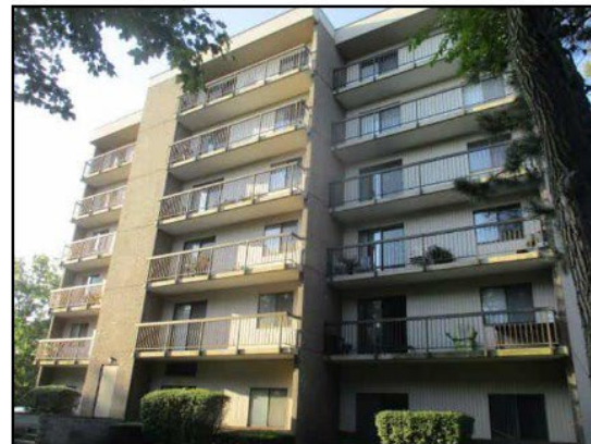
18. Back building elevation (north) facing southeast.
