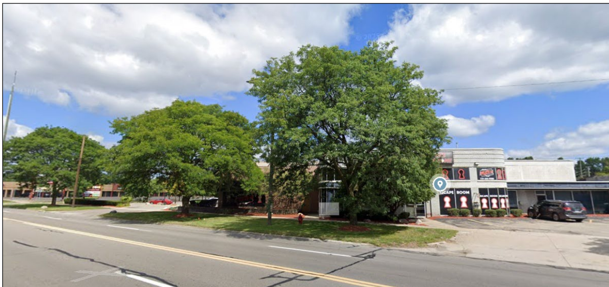
Streetview from Grand River Avenue (Google Maps Streetview 2024)
