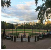
Ball Diamond Renovation
