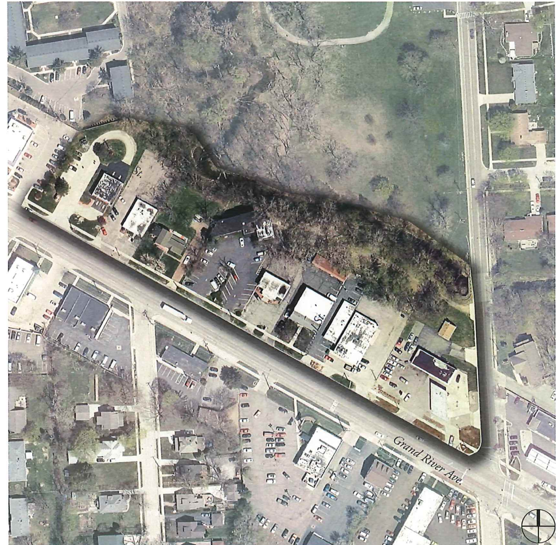
FIGURE 3.16 SUBAREA E - EXISTING CONDITION
